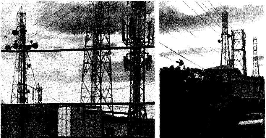
Pic no. 4 Mobile Towers
